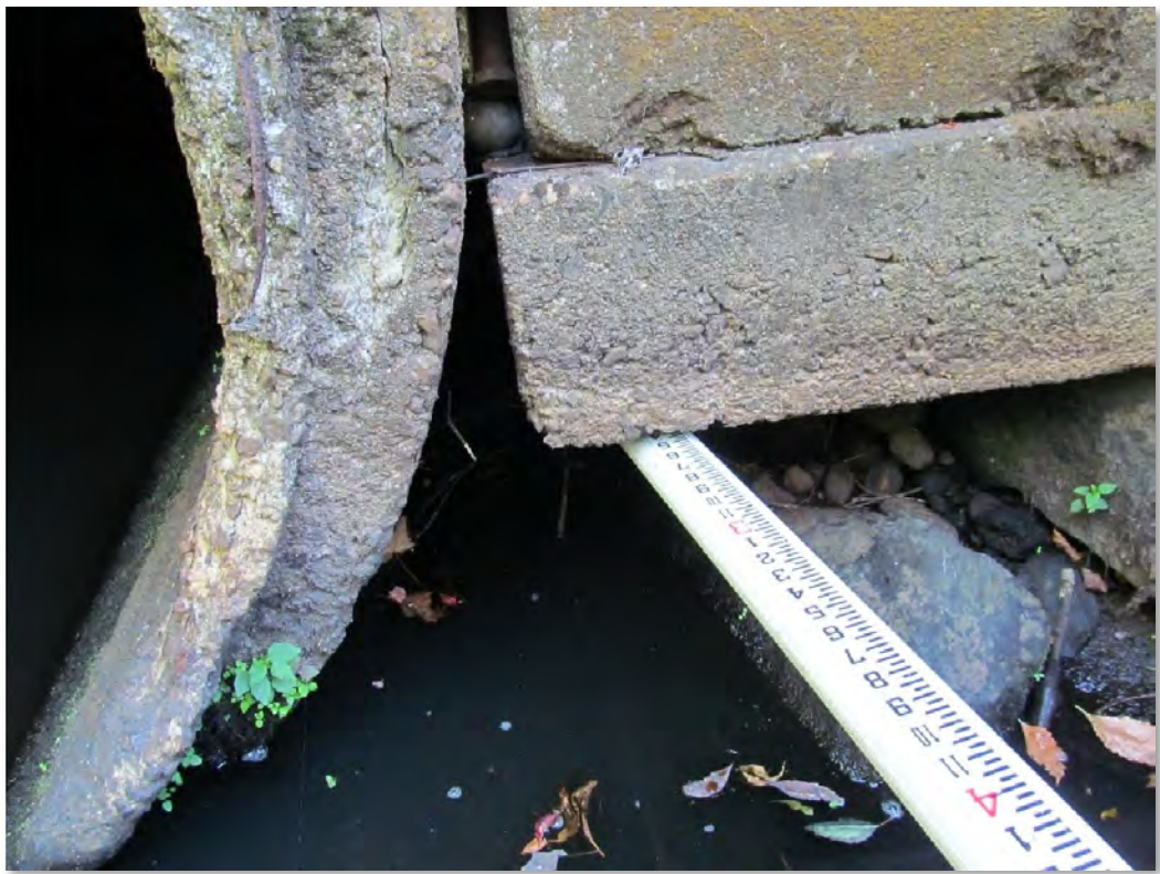
Photo 20: Southwest Corner Undermining
