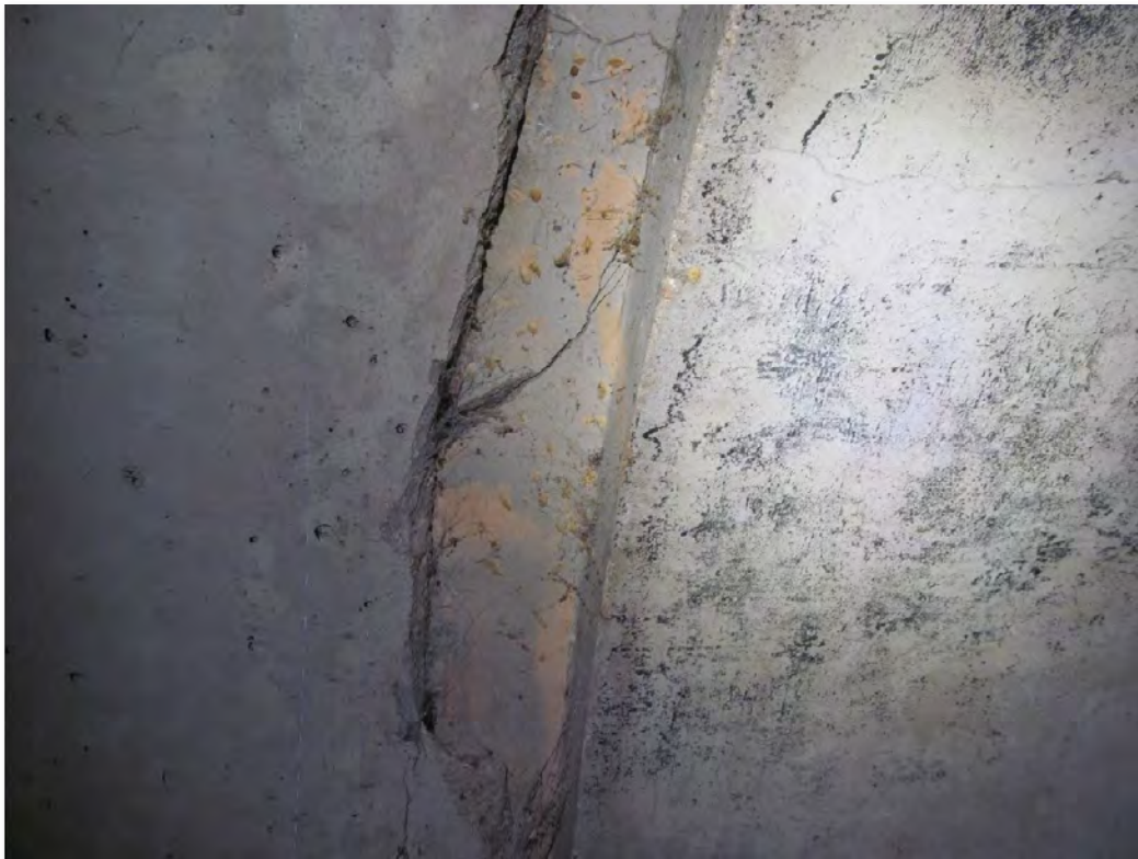
Photo 17: South Pipe, 8th Segment, Typical Cracks and Spalls in Pipe Connections
