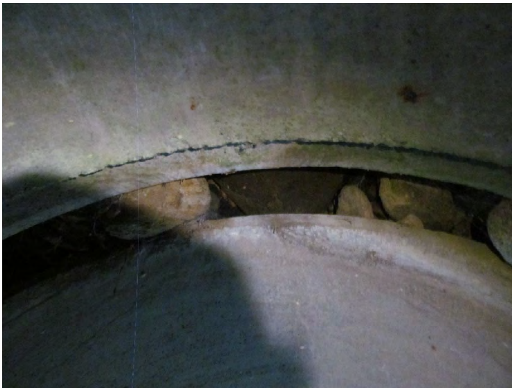
Photo 16: North Pipe Largest Gap Between Sections, West End Section
