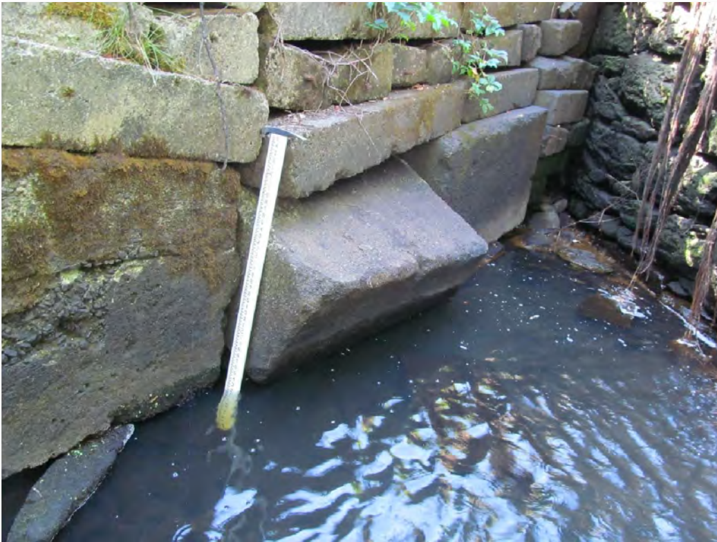
Photo 12: Southwest Embankment Wall Settled Block
