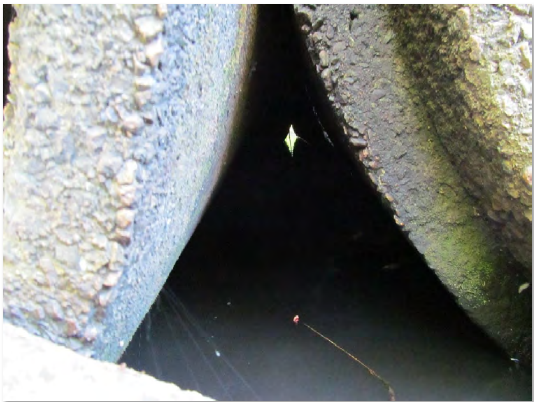
Photo 19: Gap Between South and North Pipes
