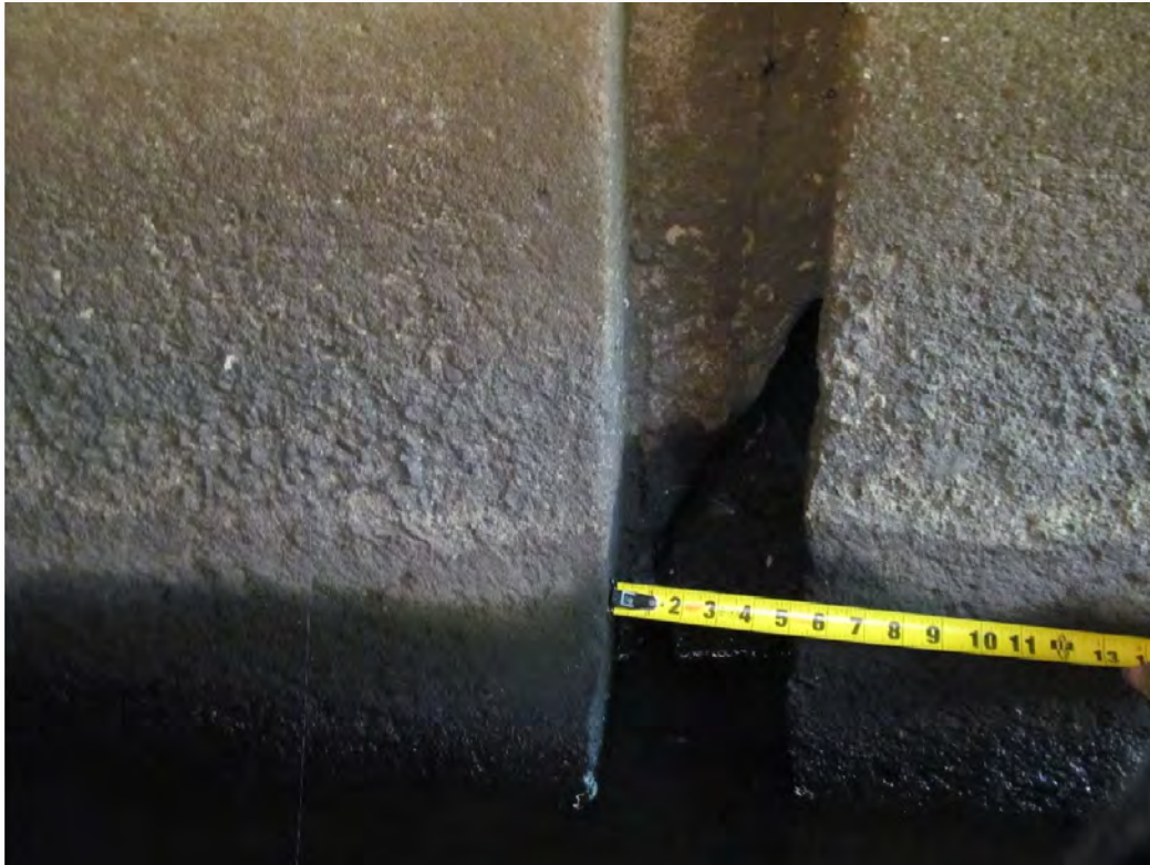
Photo 15: South Pipe Largest Gap Between Sections, East End Section
