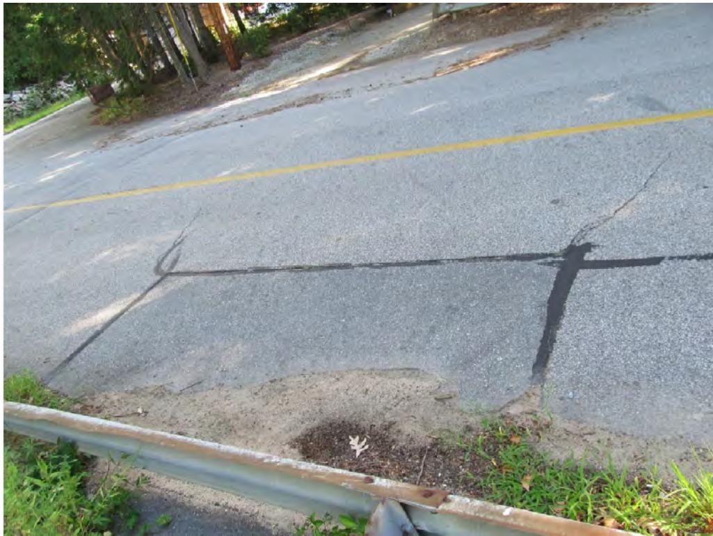
Photo 6: Patch in Wearing Surface with Associated Cracks
