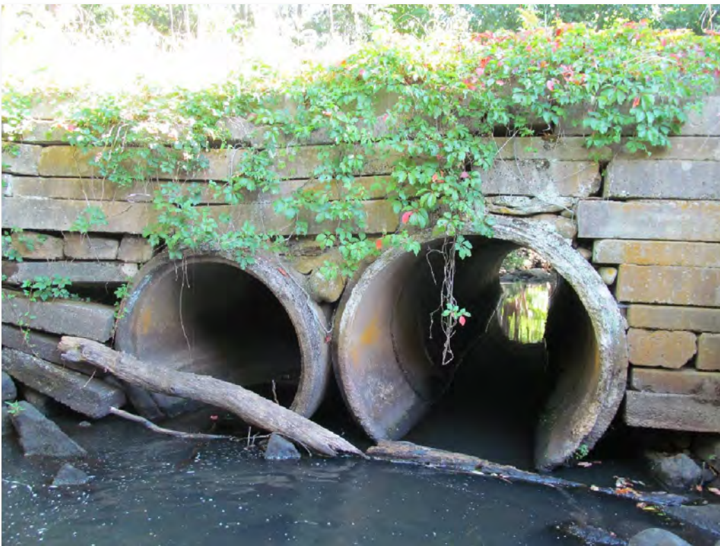
Photo 24: Logs Partially Blocking Pipe Inlets
