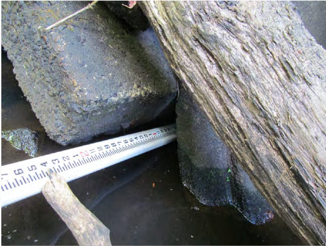
Photo 21: Northwest Corner Undermining
