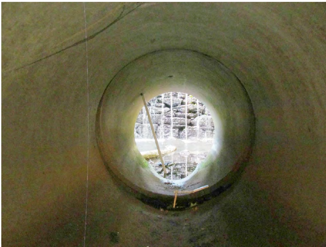
Photo 18: North Pipe West Section Settlement Blocking Water Flow
